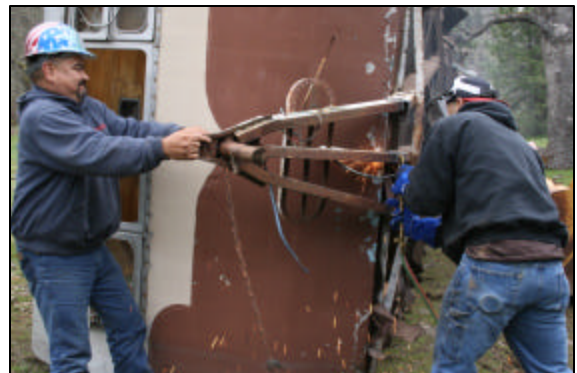
Chuck Carl tugs as J.J. Waltermann uses blow torch to disconnect the trailer hitch from the old trailer.
