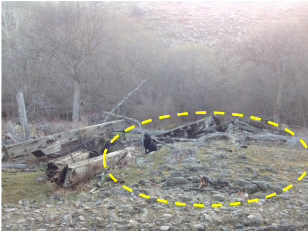
Figure 103. Remnants of bridge (left) washed-out and deposited by the 1964 flood on a high floodplain surface 1900 lineal feet down-valley (~VM 8.6). Note sediment wedge (circled) to right/upstream of bridge debris. Surface clasts wedge have dense lichen cover (right).
