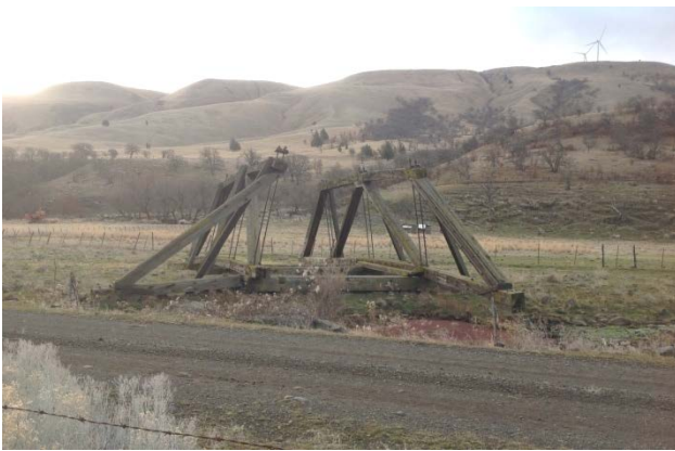
Figure 102. Bridge (left) that was washed off its piling foundation 1500 lineal feet upstream (right) and deposited by the 1964 flood on a high floodplain surface (~VM 10.1).
