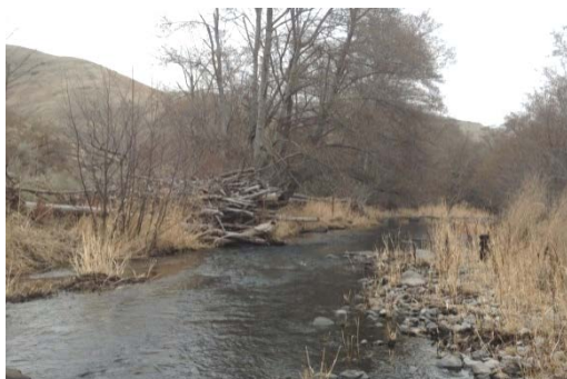
Figure 41. Example of woody debris spurs; raked into riparian trees, oriented perpendicular to channel, with one end butted into a higher topographic surface.
